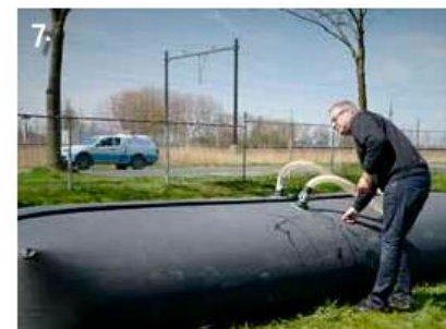
Fill the SLAMDAM® to a height of about 67 cm.
