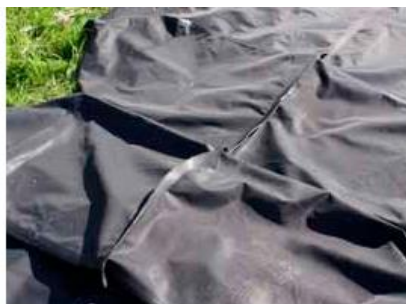
Make sure the weld on the bottom of the first SLAMDAM® follows the line of the next SLAMDAM®.
