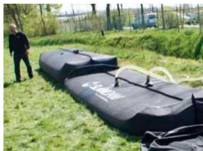
By repeating this steps, length is created by placing several SLAMDAMS in a row like a chain.
