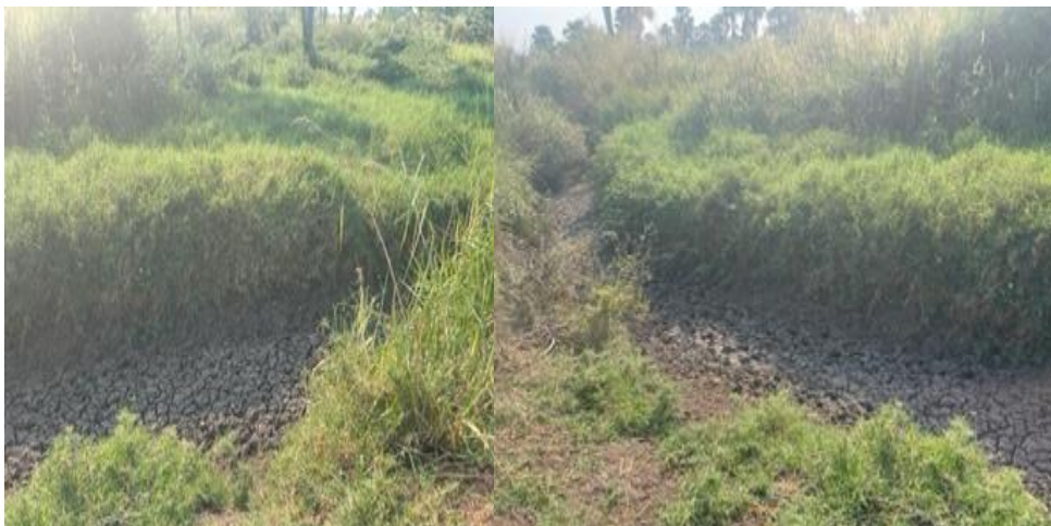
Figure 2.5: An excavated channel, constructed by the Danish Refugee Council to drain water towards the South instead of into the direction of Waka
