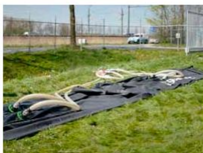
The SLAMDAM® is now ready to be filled with water. Both SLAMDAM® compartments must be filled simultaneously.
