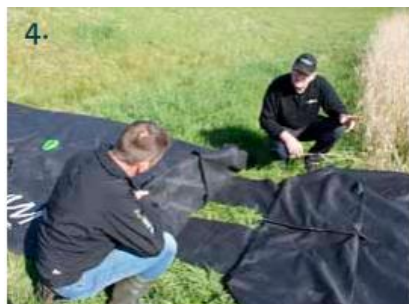
Place the next empty SLAMDAM® and follow the line of the first SLAMDAM®.
